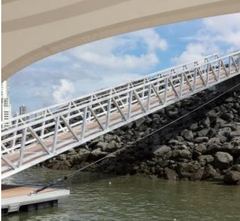
Photo from Structurmarine
