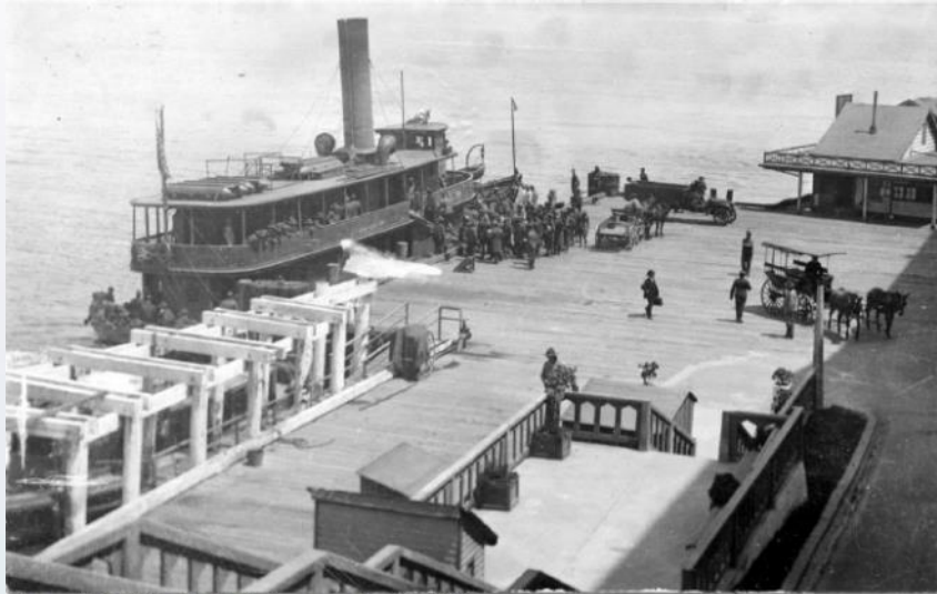
Figure 2-63. Wharf (c1919) (source: GOGA-3089)
